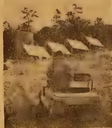
ILS solar collectors, heat storage, and "Windmule"—electric pickup.
